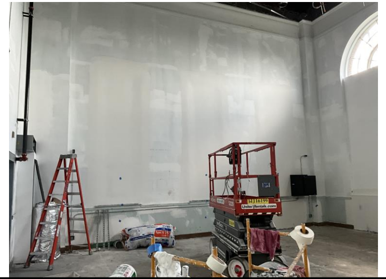
Dance studio construction at Hope High School
