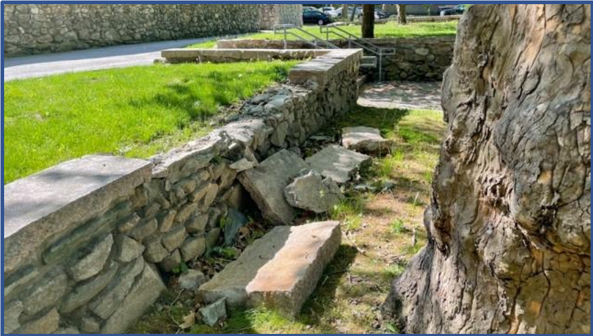
Masonry Repairs at MLK (Before)
