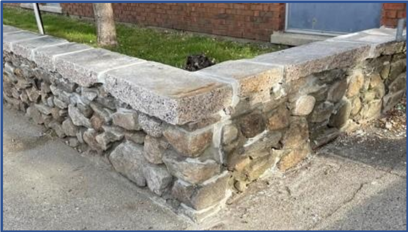
Masonry Repairs at MLK (After)
